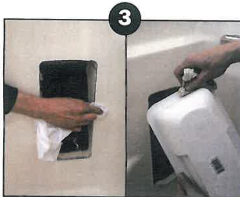
It is very important to clean the area around the cut out with an alcohol solvent. The flange on the stowagebox should also be cleaned.
